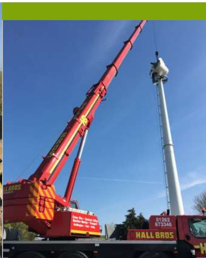
The nacelle is gently lowered onto the tower and fixed in place
