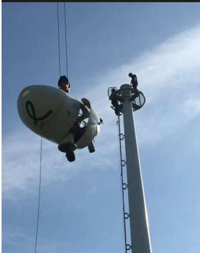
The nacelle is craned back on to the tower
