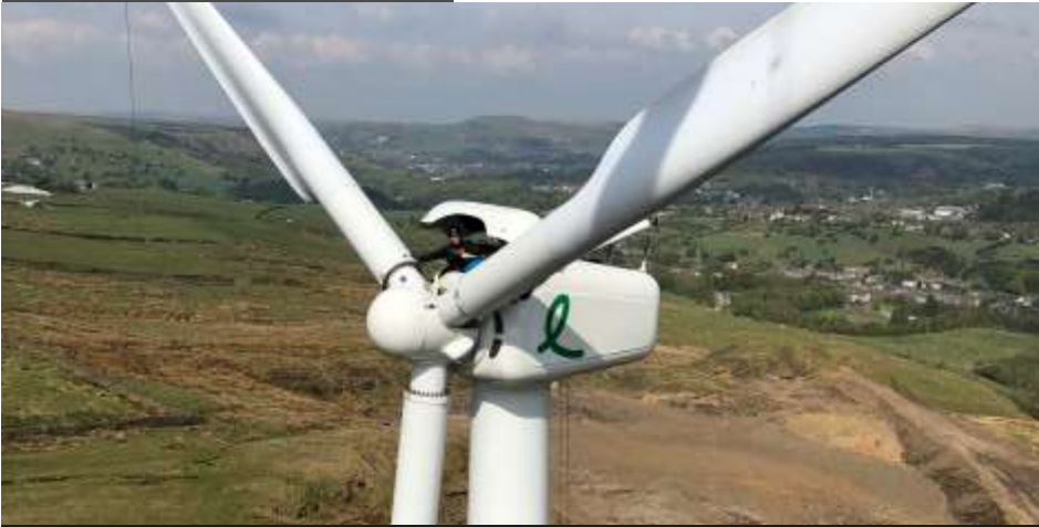
The first refurbished X35 nacelle being installed in Lancashire
